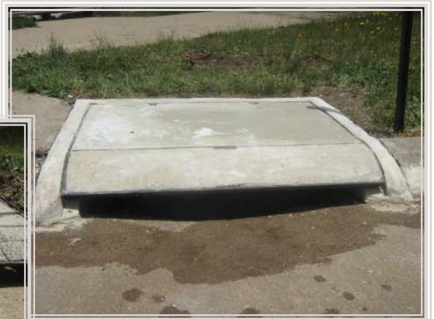
Pit after repair
