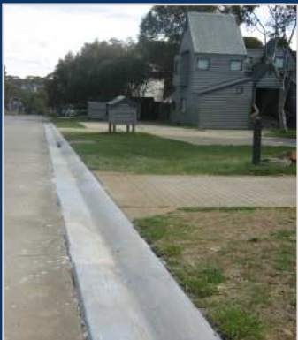
Kerb after repair
